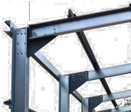
SS Steel posts and beams (exposed) Colour: Galvanised - zinc
